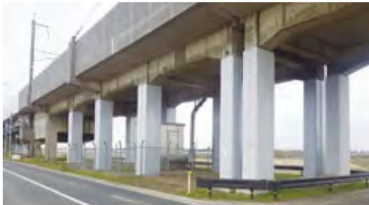
Seismic reinforcement of elevated railway tracks
