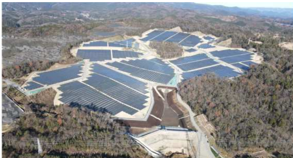
Image-2 Project SE-02 Isohara Extra-high Voltage Power Plant, Kitaibaraki, Ibaraki
