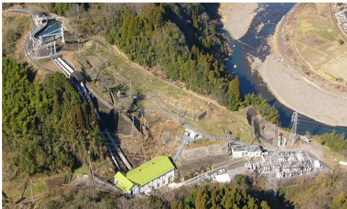
Photo-2 Hydroelectric power generation business Jikumaru power station * Before renewal work
