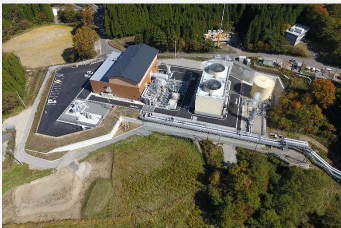
Photo-3 Geothermal power generation business Otake power station * After renewal work
