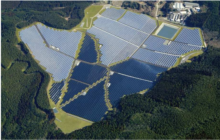
Project 01 Ashikita Solar Power Station, Solar PV
