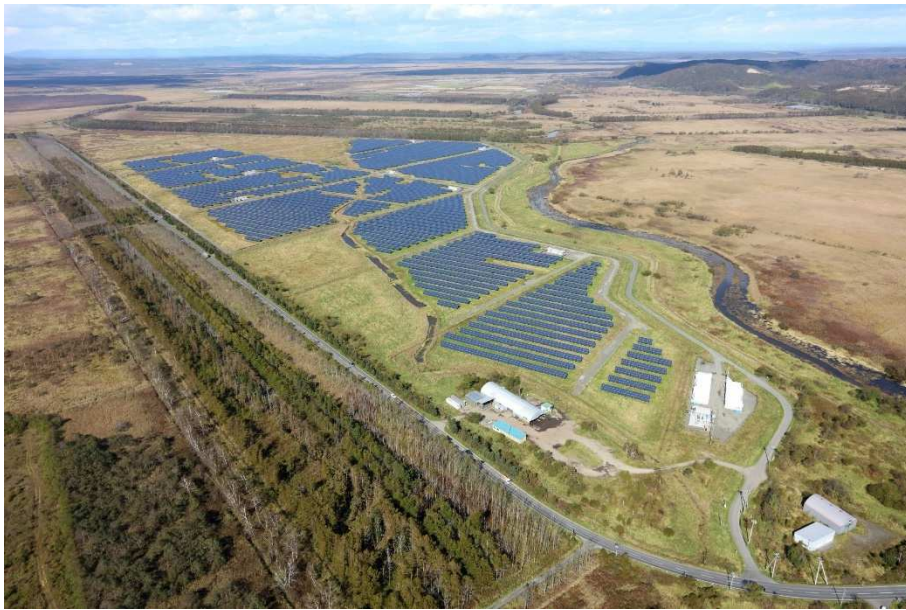
Project 02 Kushirocho Toritoushigenya Solar Power Station, Solar PV
