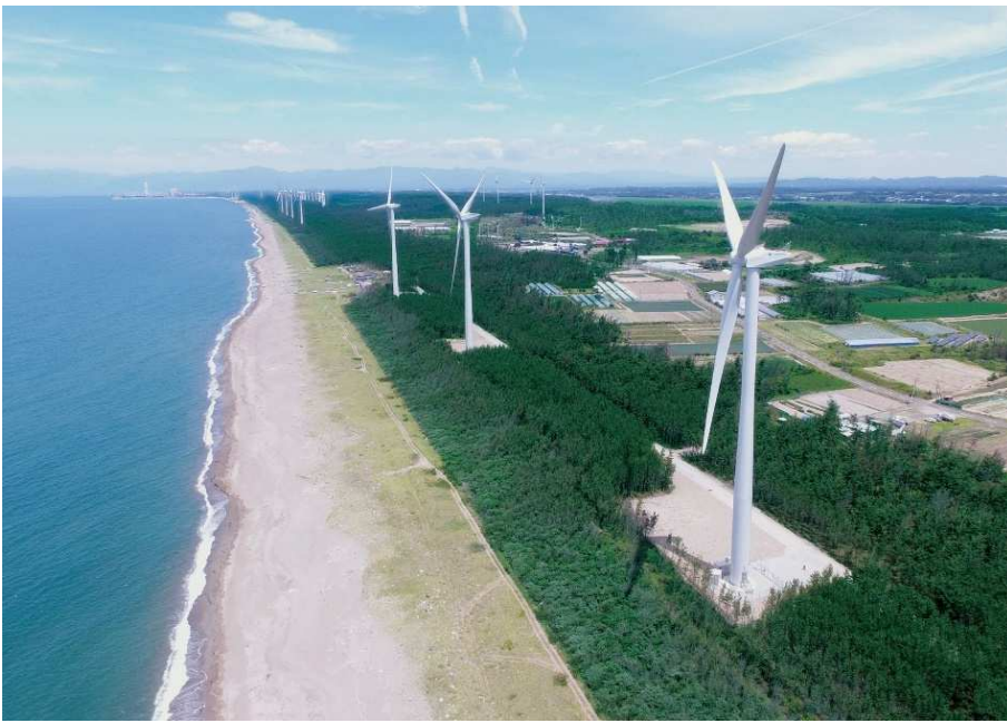
Project 04 Mitanehamada Wind Power Station
