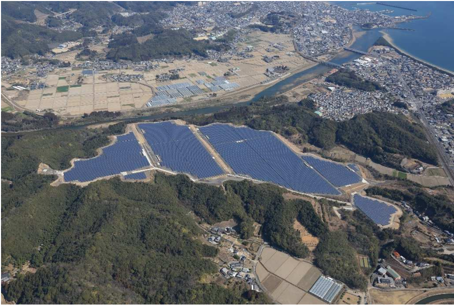
Project 03 Hyugahichiya Solar Power Station, Solar PV
