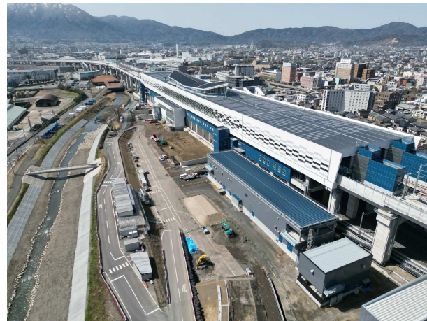
Exterior view of Tsuruga Station #1 (Fukui Prefecture)
