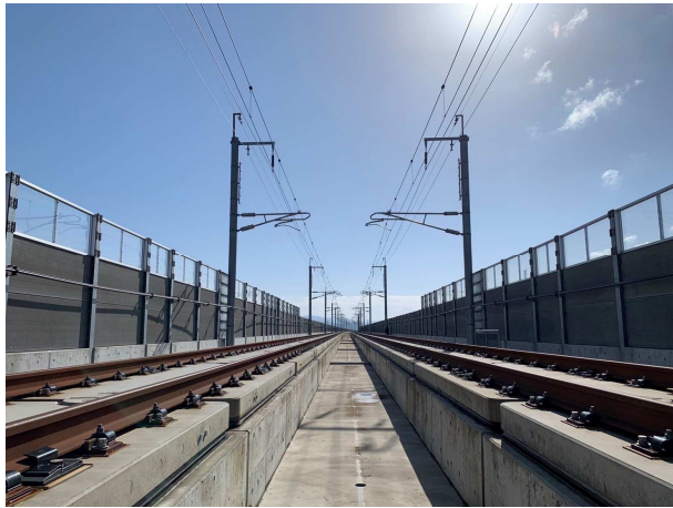
Interior view of viaduct (Fukui Prefecture)
