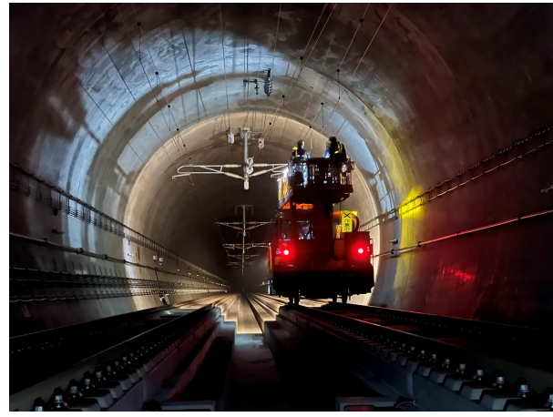
Interior view of Tunnel (Fukui Prefecture)
