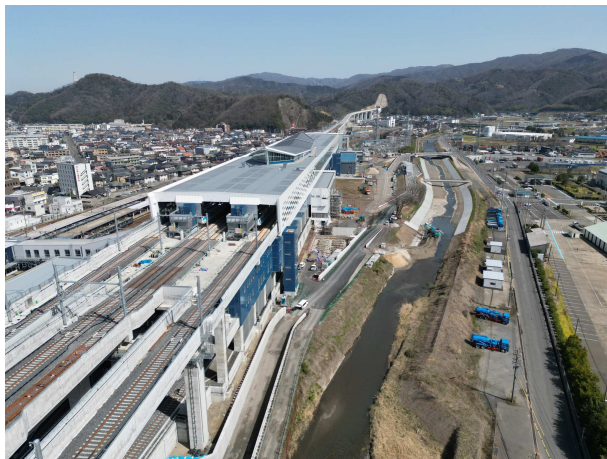
Exterior view of Tsuruga Station #1 (Fukui Prefecture)
