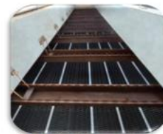
Inclined Plate Sedimentation System
