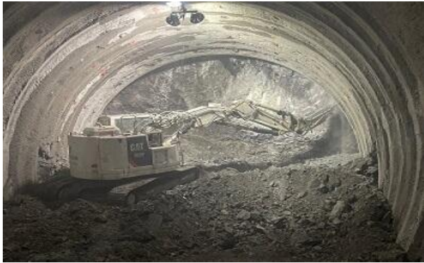
Oshima Tunnel (Minamiuzura) (Hokuto, Assabu) Under tunnel excavation
