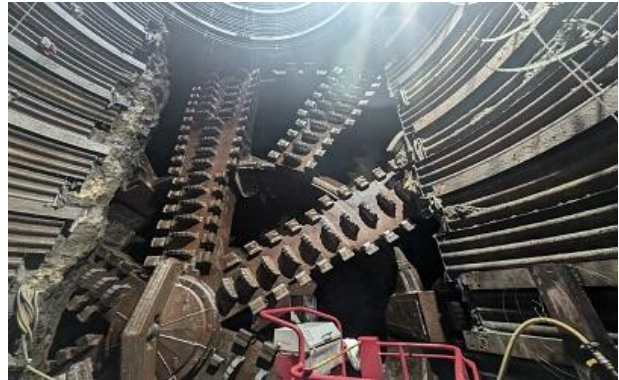
Yotei Tunnel (Hirafu) (Niseko, Kutchan) Intermediate vertical pile machine faceplate
