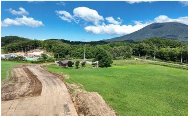
Yotei Tunnel (Arishima) (Niseko) Above ground
