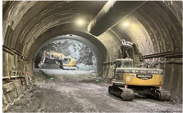
Oshima Tunnel (Daibayama) (Hokuto) Under tunnel excavation
